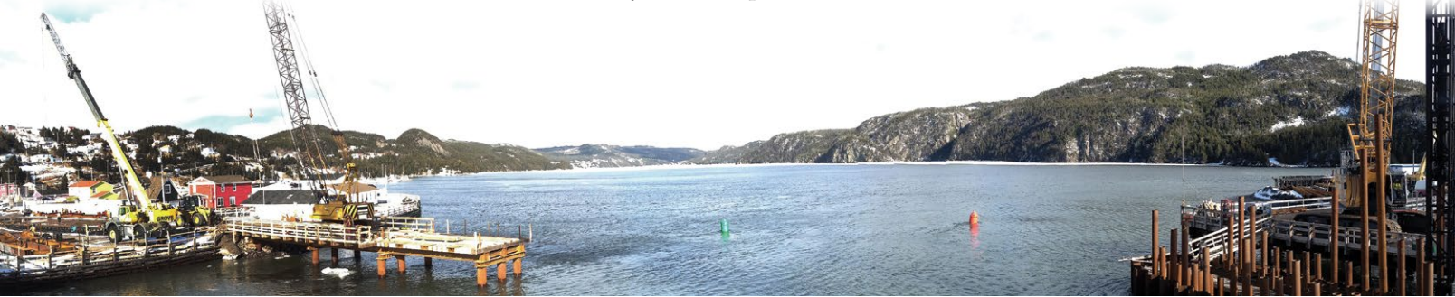
COURTESY OF H.J. O'CONNELL-VANCOUVER PILE DRIVING JOINT VENTURE
