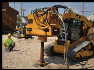
Ready for low overhead work.
