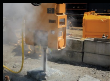
Setup for Down Hole Hammer.
