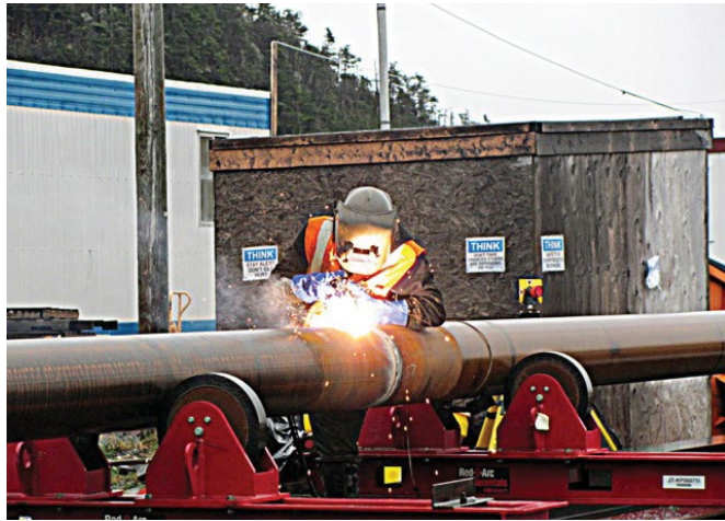
December 4, 2013 – Splicing 12.75-inch pipe piles on the welding bed
