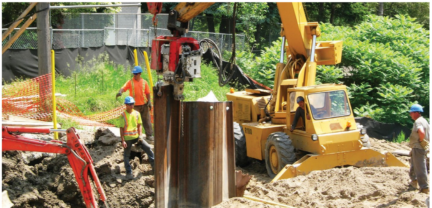
Dawson excavator mounted vibro
